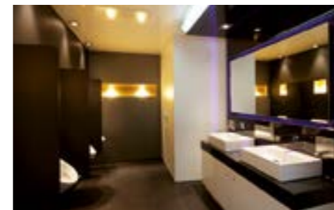
KITCHEN & SANITARY INSTALLATIONS
