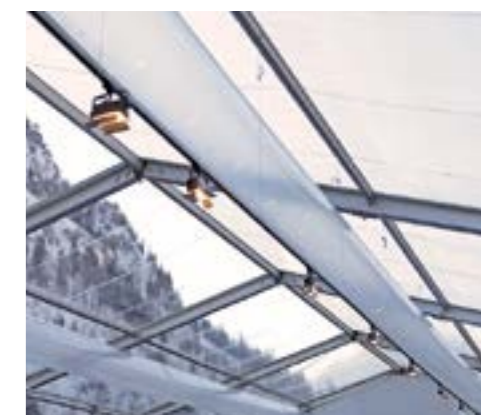
HEATING & AIR CONDITIONING SYSTEMS
