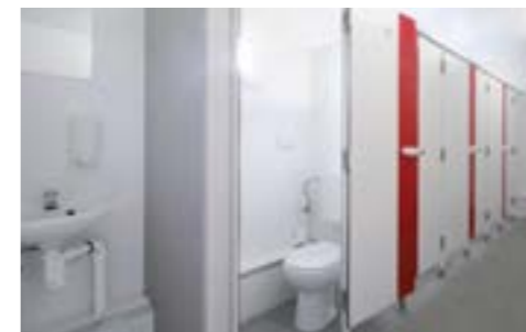
KITCHEN & SANITARY INSTALLATIONS
